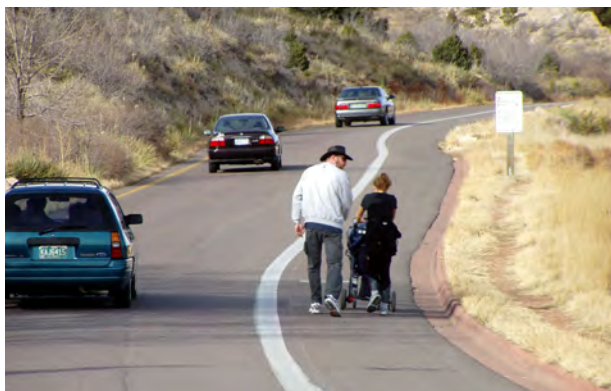
Paved shoulder used as a walkway.
