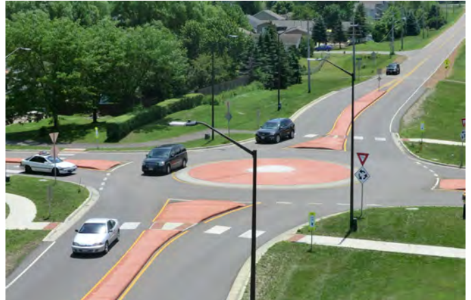
Example of a single-lane roundabout.
